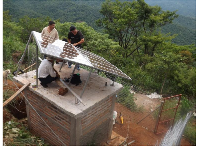
Installing solar panels on the depot
